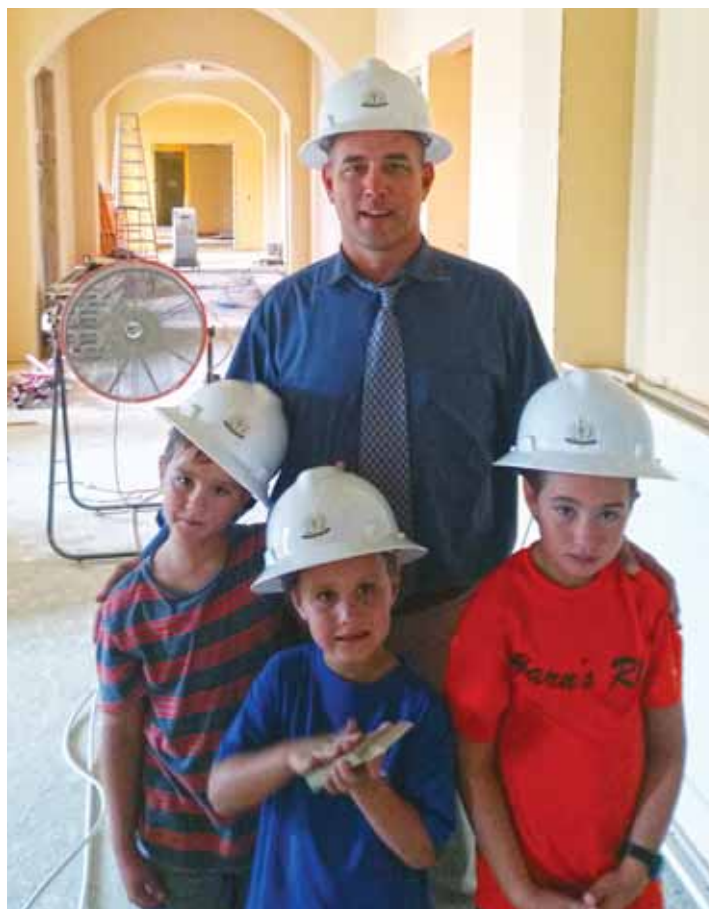
The third generation of the privately owned Caldwell Trust Company takes a hard-hat tour of the new headquarters with their father, R. G. “Kelly” Caldwell, Jr., CEO and president, in late August 2014. The boys (Zachary, 8; Chase, 5; and Brooks, 9) were onsite just three months before the company took up residence.
